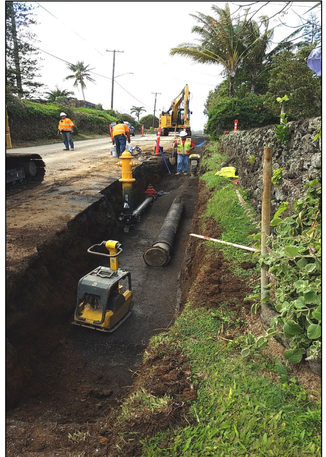
Crews work installing a new 12-inch waterline and fire hydrant along Akoni Pule Highway (Hwy. 270). Photo credit: DWS.
