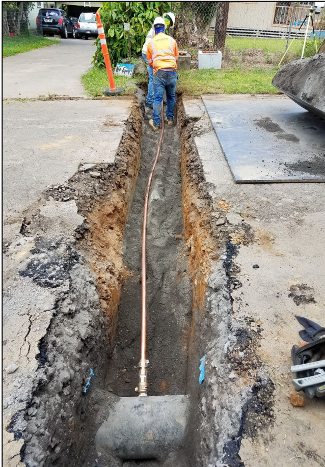
A new service lateral will deliver safe drinking water to a customer's home on Ma'ulili Road. Photo credit: DWS.
