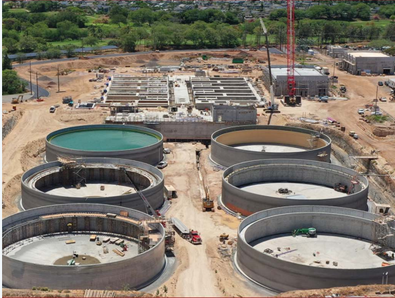
Tank Project: 6 x 2.0 MG Clarifiers — Honolulu WWTP
